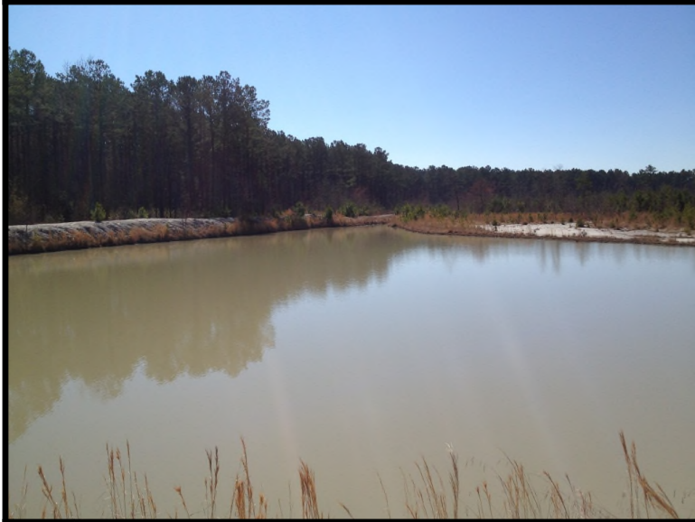
9 Upland-dug detention pond located on the western portion of the site.
