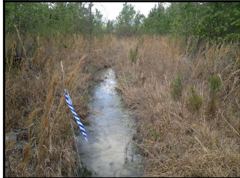
8 Non-jurisdictional linear conveyance (NJLC-2) located on the southwestern portion of the site.
