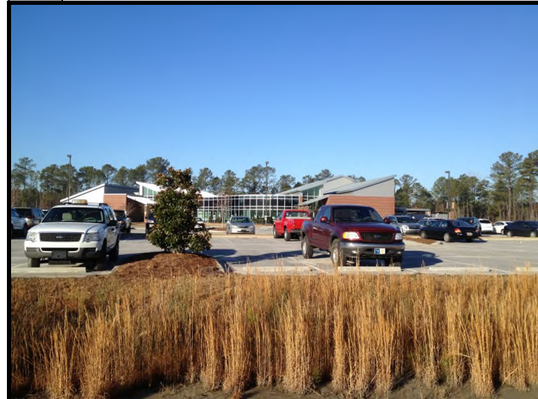
4 County building currently occupied by the Kershaw Campus of Central Carolina Technical College and the Kershaw County Economic Development Office.
