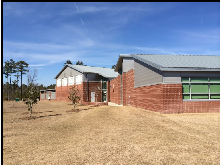
3 County building currently occupied by the Kershaw Campus of Central Carolina Technical College and the Kershaw County Economic Development Office.
