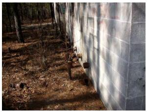
Photo #11 Chemical drain pipes protruding from Wateree Chemical building
