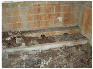
Photo #12 View of chemical collection trough with drains inside Wateree Chemical building.
